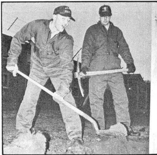
(photo, top left) CTM2 Bradley Nielsen breaks up the concrete around a post. (top right, from left) CTM2 James Brooks and CTR2 Jason Todd dislodge a post. (bottom, from left) CTM3 Chris Davenport and CTR1 Dave Ward loosen the ground around another post.
